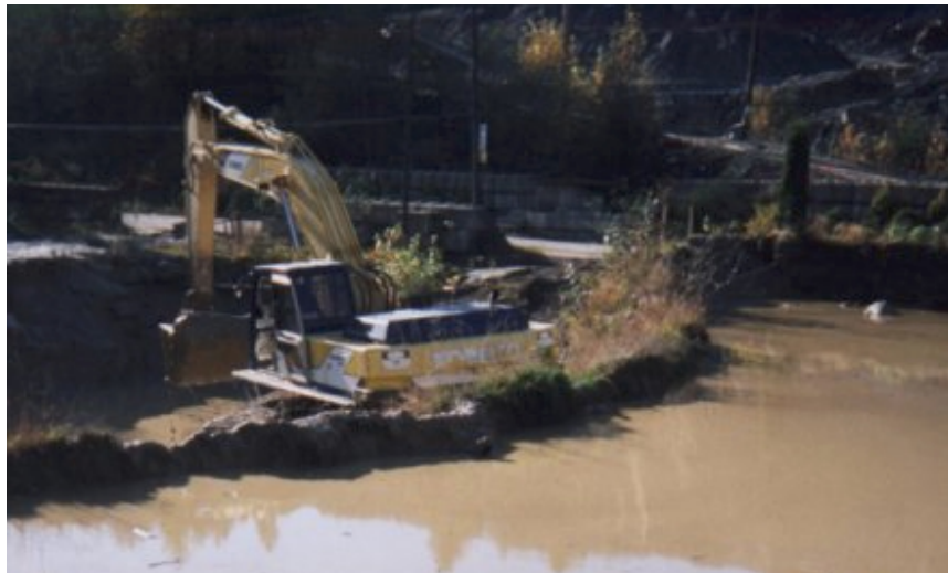
Cleaning a settling pond at an aggregate mining operation
